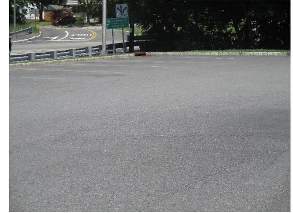
Parking spaces west of the building can be replaced with porous asphalt to infiltrate stormwater. A preliminary soil assessment suggests that more soil testing would be required before determining the soil's suitability for green infrastructure.
