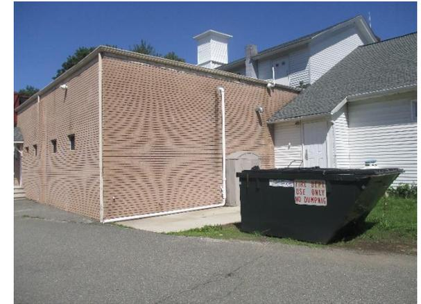
Parking spaces on the north side and west side of the building can be replaced with porous asphalt to infiltrate stormwater. Rainwater can be harvested by installing a cistern at the southwest corner of the building and be used for washing trucks. A preliminary soil assessment suggests that the soils have suitable drainage characteristics for green infrastructure.
