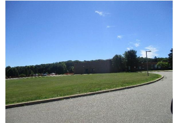
The basketball court and parking spaces in the lot south of the building can be replaced with porous asphalt to infiltrate stormwater. A rain garden north of the building can capture, treat, and infiltrate roof runoff. A preliminary soil assessment suggests that the soils have suitable drainage characteristics for green infrastructure.
