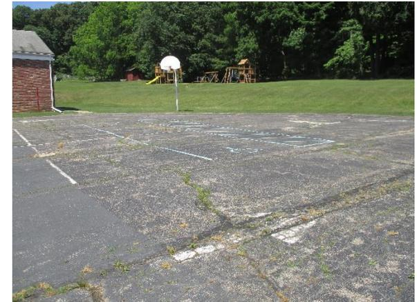
Parking spaces northwest of the building can be replaced with porous asphalt to infiltrate stormwater from the roof and parking lot. A preliminary soil assessment suggests that the soils have suitable drainage characteristics for green infrastructure.
