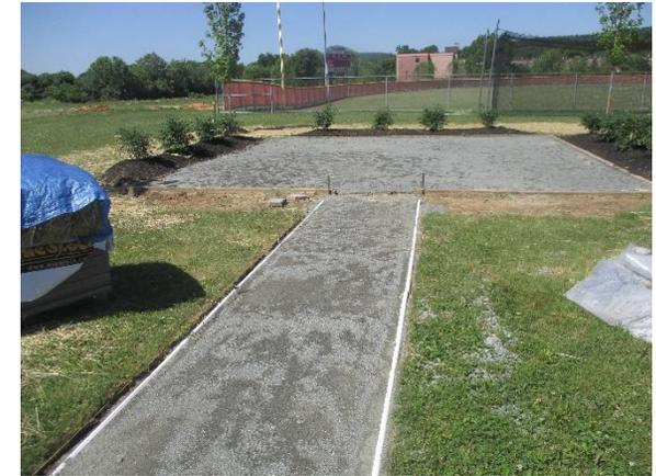
Parking spaces and the basketball court can be replaced with porous asphalt to infiltrate stormwater. A preliminary soil assessment suggests that more soil testing would be required before determining the soil's suitability for green infrastructure.
