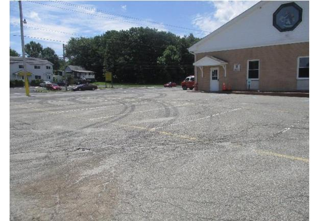
Parking spaces north and east of the building can be replaced with porous asphalt to infiltrate stormwater. Rainwater can be harvested by installing a cistern at the northeast corner of the building for washing trucks. A preliminary soil assessment suggests that the soils have suitable drainage characteristics for green infrastructure.
