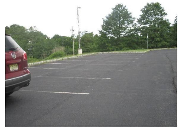
Parking spaces on the east and west sides of the building can be replaced with porous asphalt to infiltrate stormwater. A preliminary soil assessment suggests that the soils have suitable drainage characteristics for green infrastructure.
